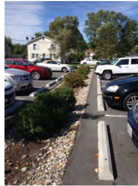
4 – Medicine Shop Infiltration Facility
