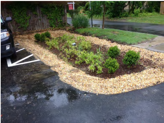
Bio-retention @ parking lot behind Carpenter Street Saloon
