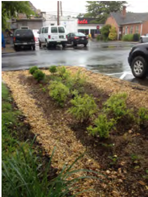
3 – Carpenter Street Infiltration Facility
