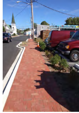
2 – ACME Market Bio-Retention
